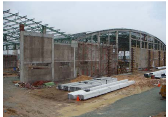
Above can see the full scale of the roof height
